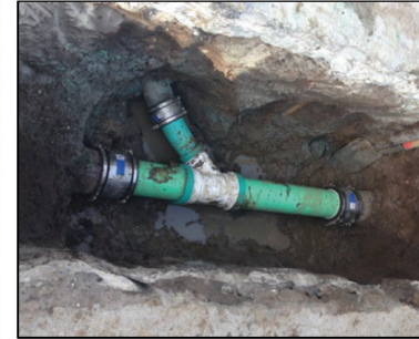
Pipe Spot Repairs
