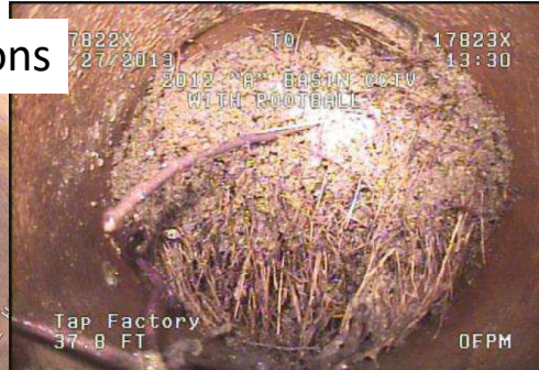
Root Intrusion in Pipe
