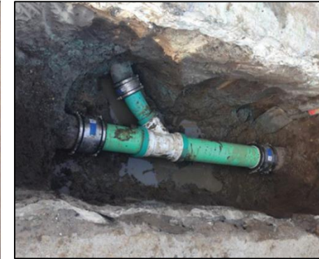
Pipe Spot Repairs
