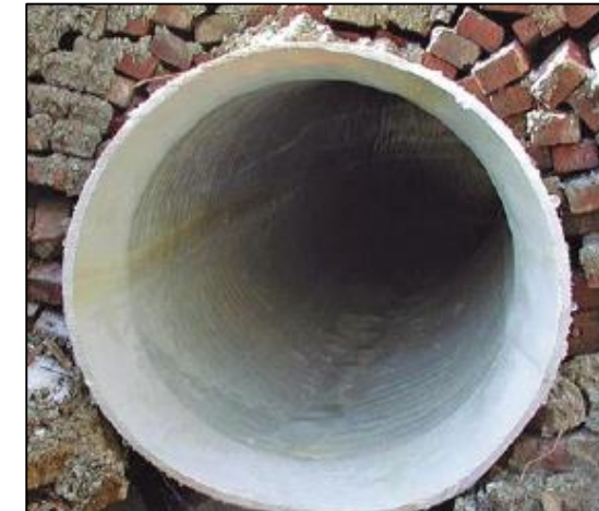
Pipe Spot Repairs
