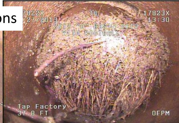
Root Intrusion in Pipe
