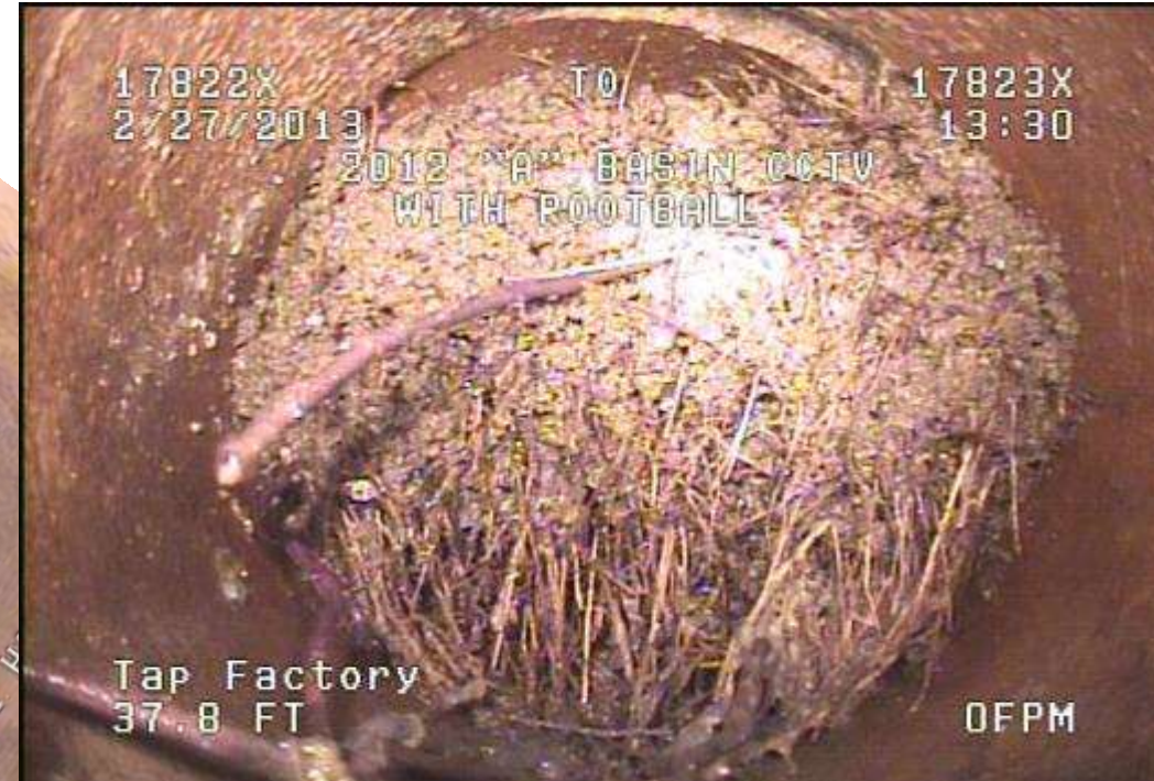
Root Intrusion in Pipe
