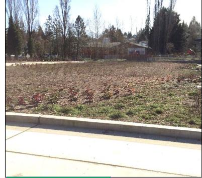
Site restored with topsoil and grass over tank
