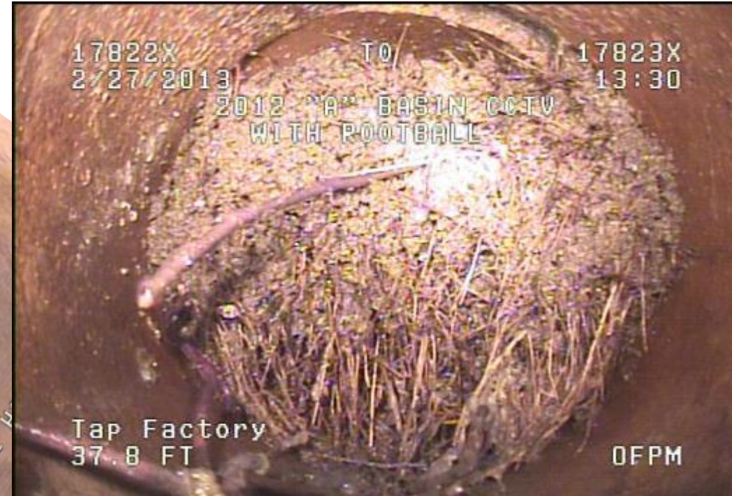
Root Intrusion in Pipe
