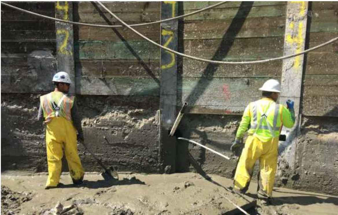
PHOTOGRAPH 6.2.2.1-2: Installation of tieback anchors within a soldier pile and lagging shoring system.
