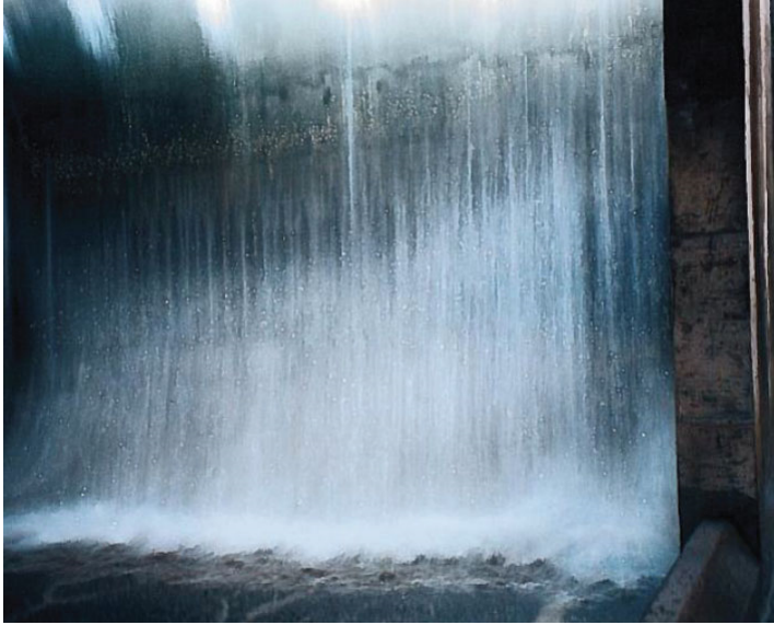
Tipping buckets flush solids and debris from holding structure to pumping system for removal
