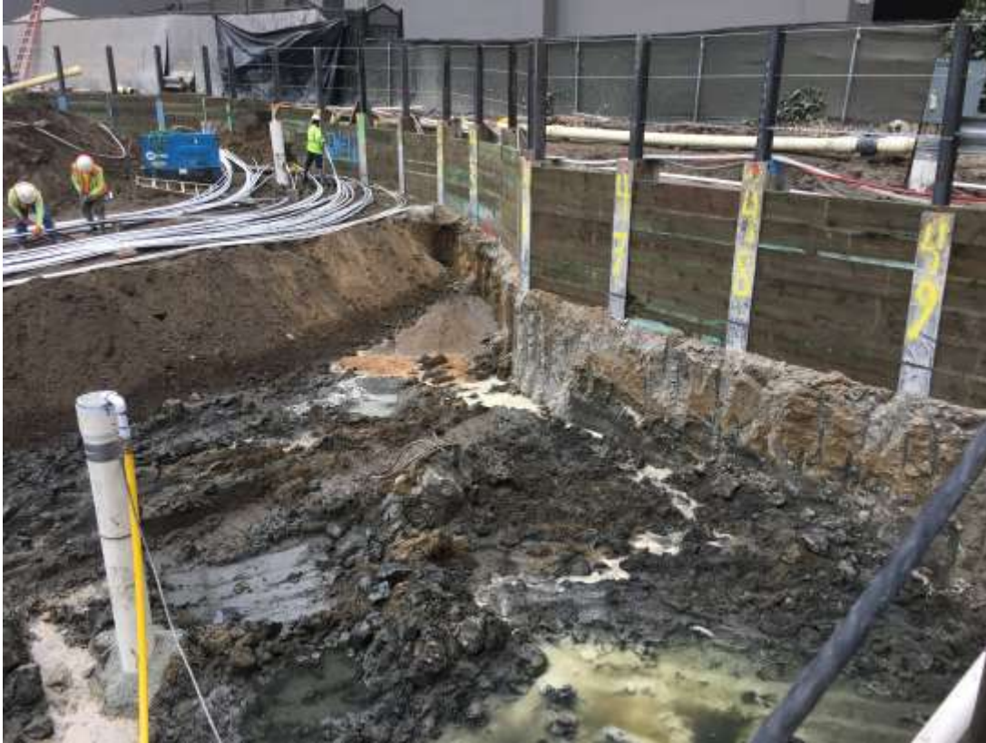
PHOTOGRAPH 6.2.2.1-1: A soldier pile and lagging shoring system with tieback anchors for a 55 feet deep excavation in San Francisco. CDSM columns were pre-installed to control water inflow. Interior dewatering wells are installed within the excavation to keep the excavation dry.
