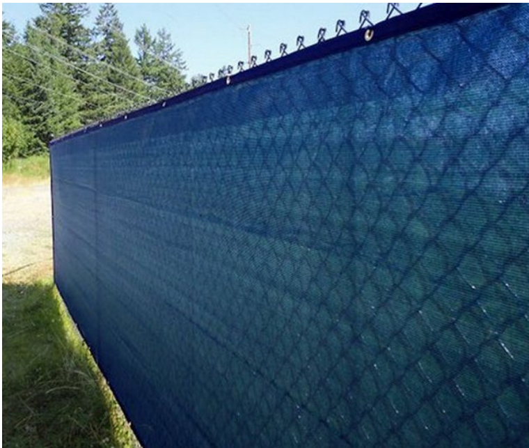
6 to 8 ft High Chain Link Fence w/ Fabric Mesh Screening
