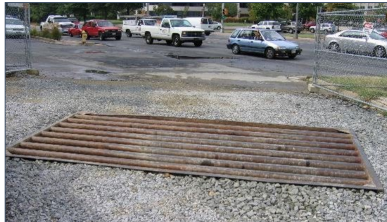
Covered Trucks, Site Watering, and Rumble Strips
