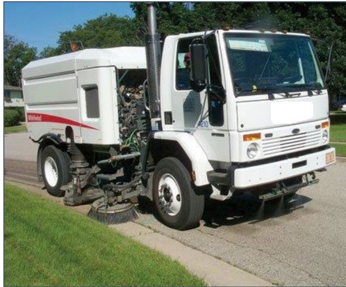
Wet Sweeping on Detroit Dr & 3 rd Ave around Construction Site
