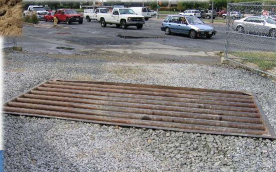
Rumble Strips at Construction Site Exits
