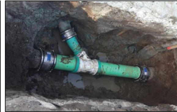
Pipe Spot Repairs
