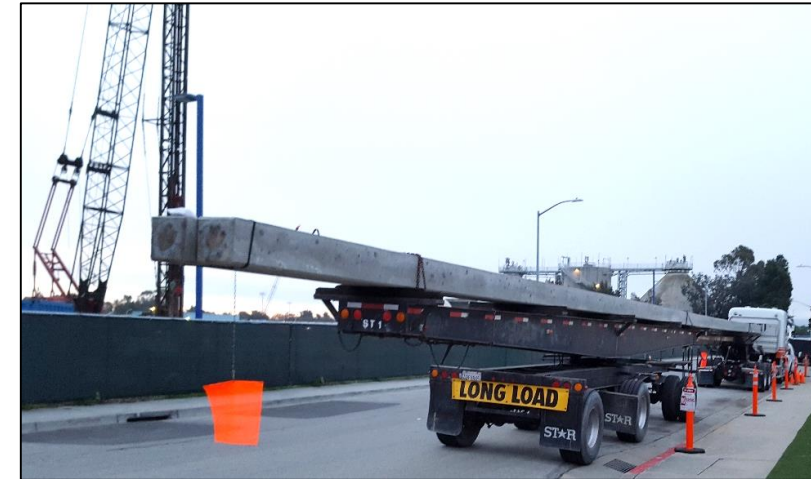
Truck Delivering Piles During On-Site Test Pile Driving (2017)
